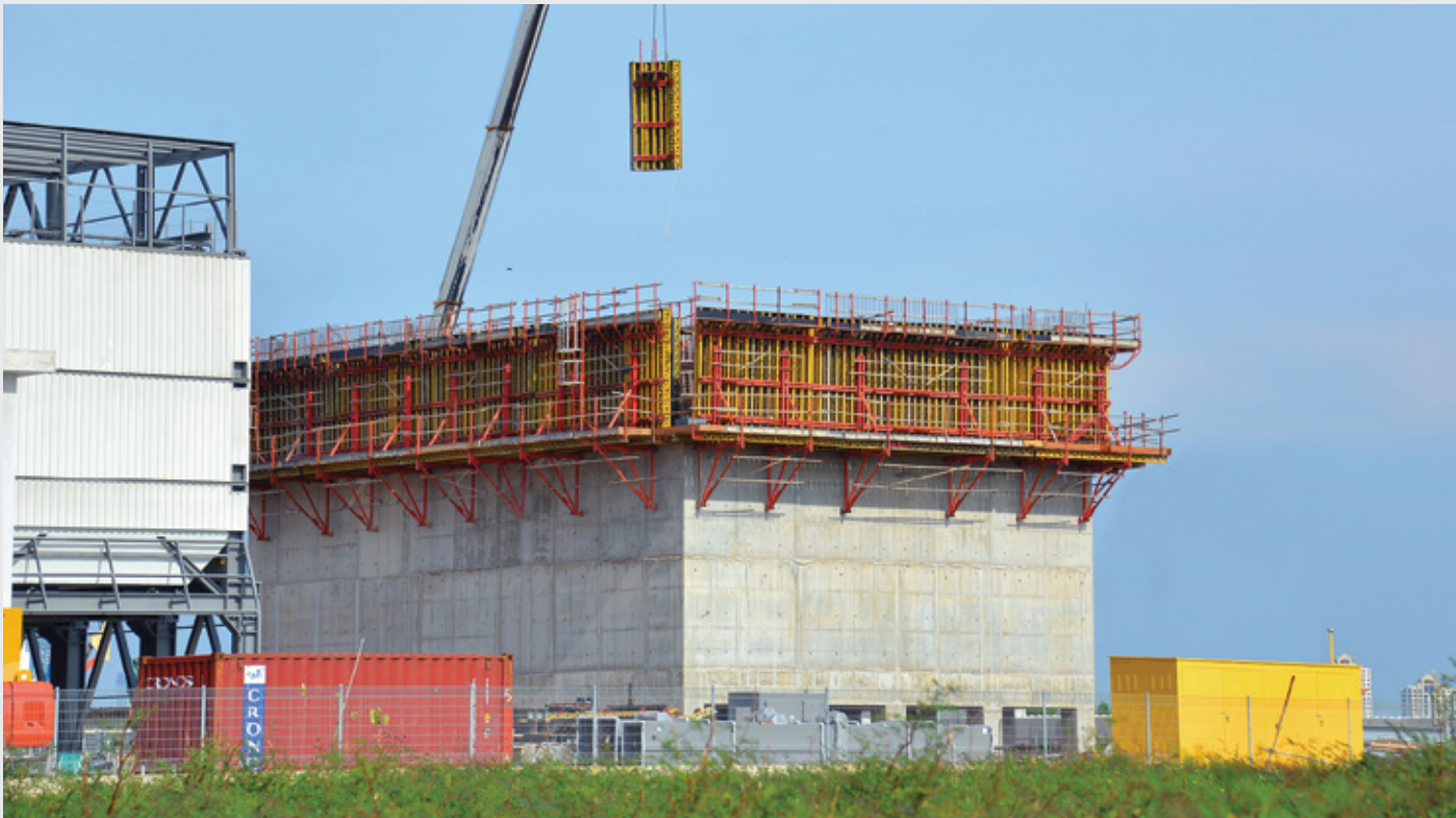
VARIO GT 24 Girder Wall Formwork in action
