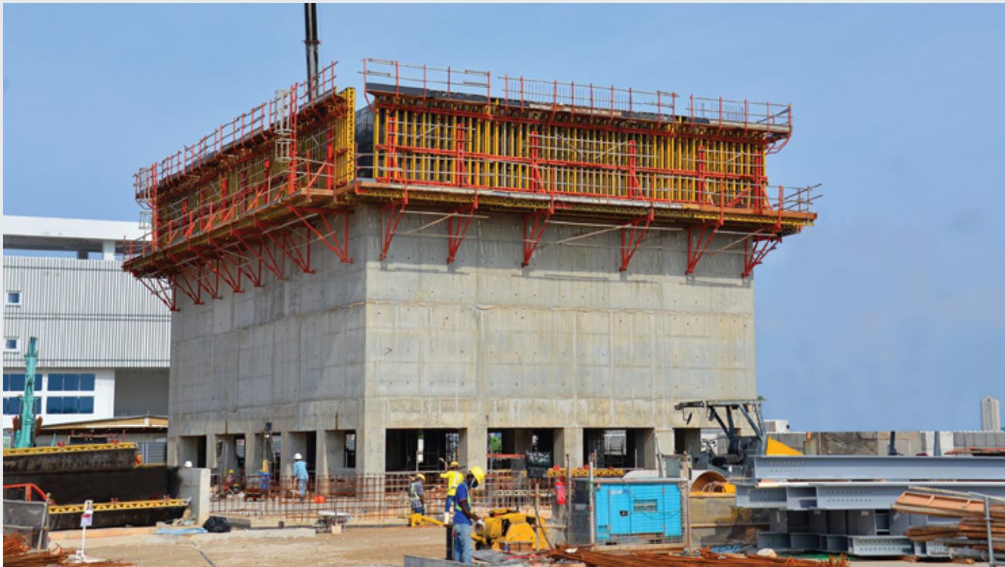
VARIO GT 24 Girder Wall Formwork in action
