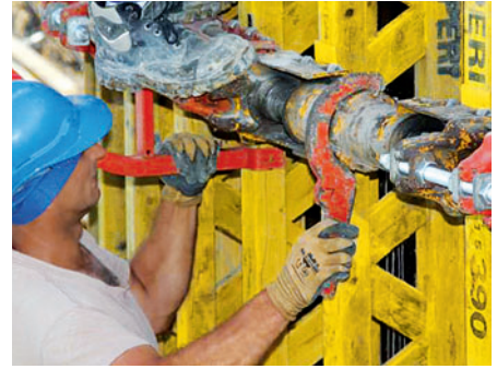
Adjusting the Articulated Spindle Waler GSRV with the Hook Spanner.
