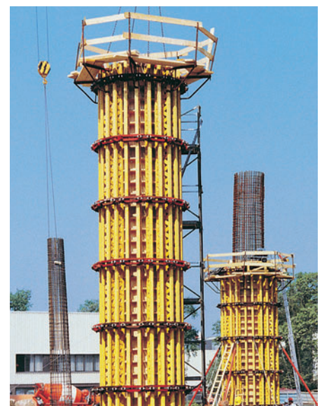
GRV in use as tapering circular column formwork.
